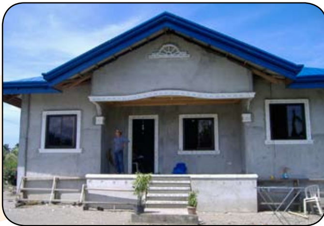
After meeting basic needs such as food, electricity and education, migrants often invest in the construction of new homes or the purchase
